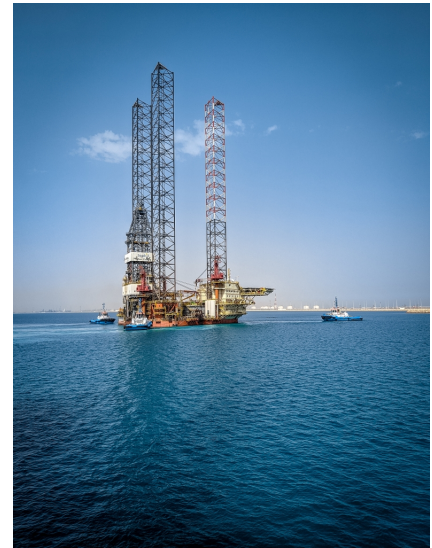
Oil rig structure that could benefit from this NASA vibration damping technology.
